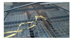
3. Once the sheild is unbolted raise the shield up to the grate and secure in place.
